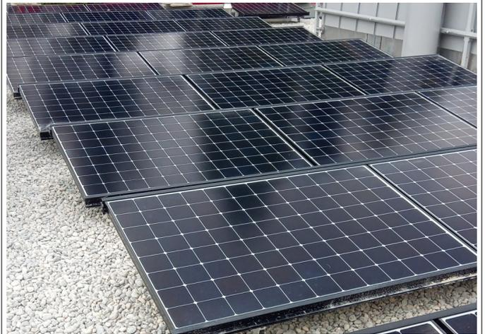
11.1 kW PV-Anlage, Sunpower 370 Watt, Montagesystem LEC-Quer, Solaredge-Optimier/Modul, Erlenbach
